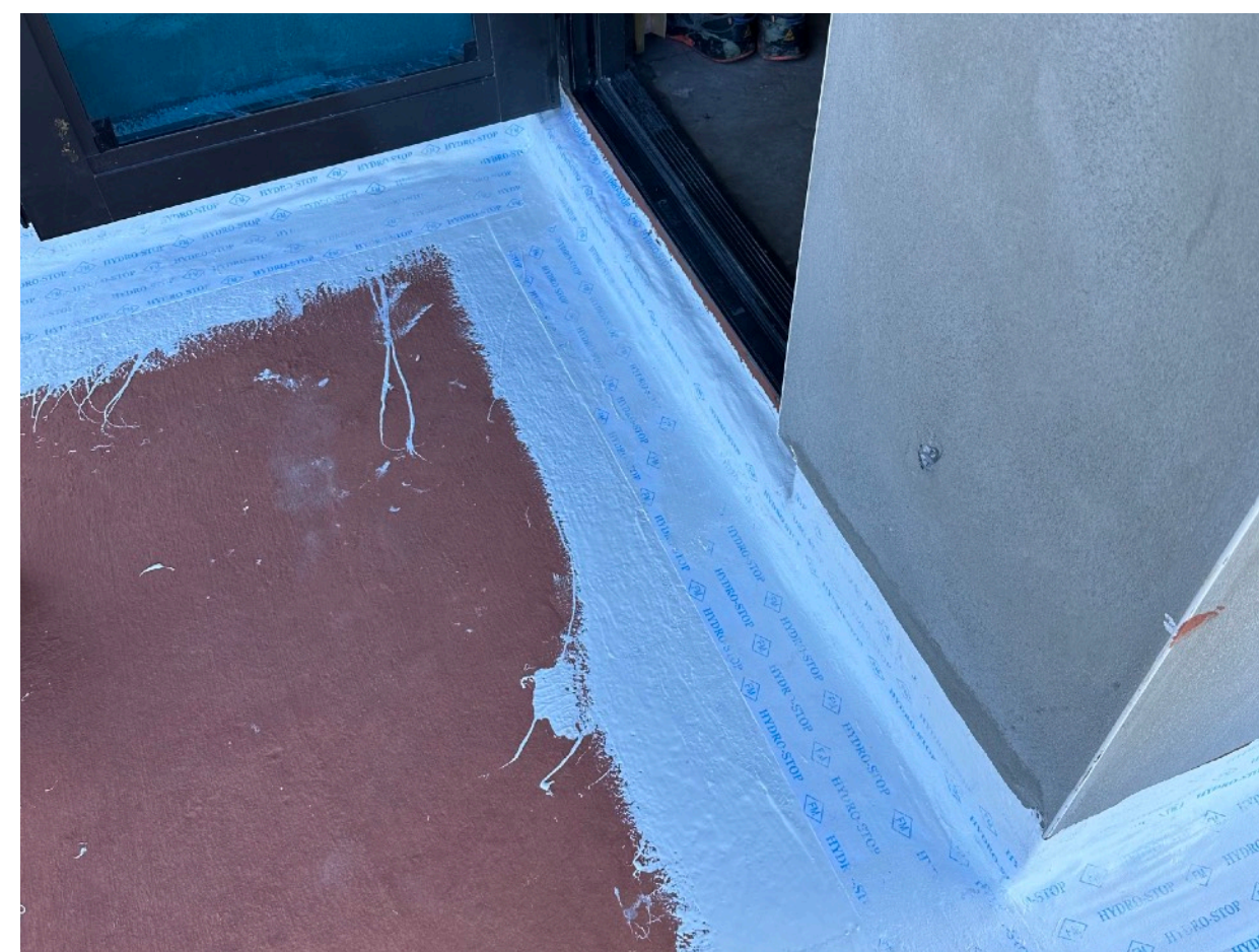
Fabric Reinforced Flashing Details
