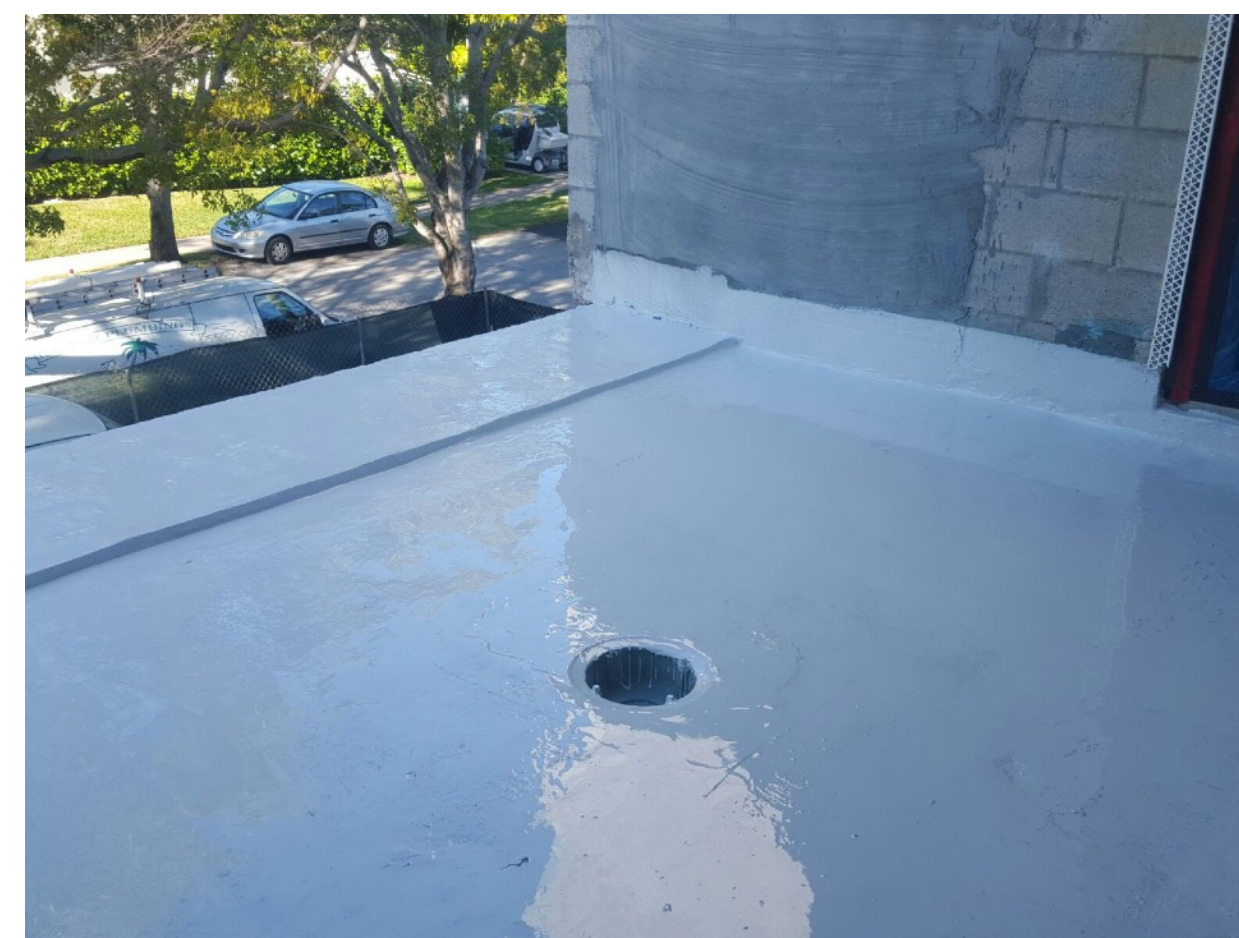
Surface Seal SB Application
